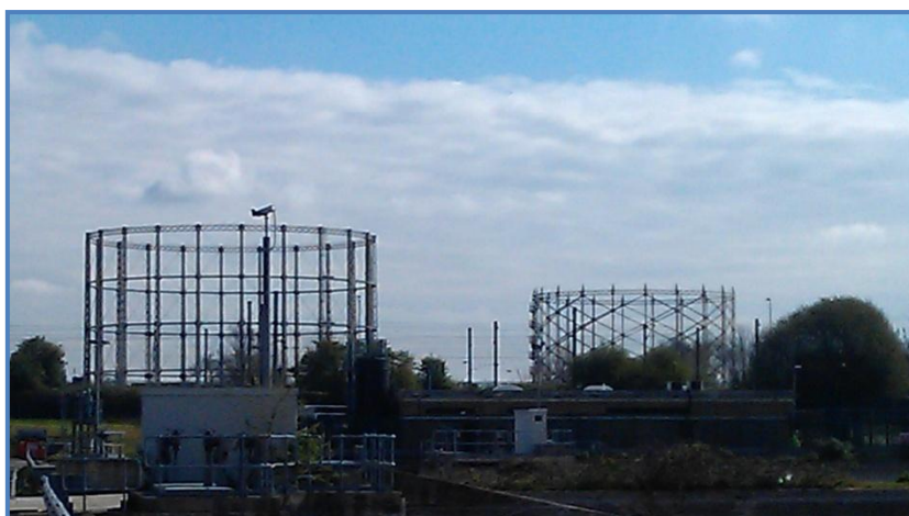
Only the gasholder on the left currently remains
